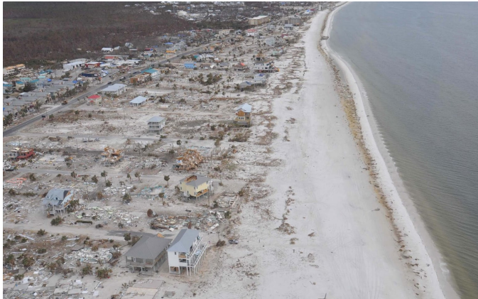
Mexico Beach – Hurricane Michael 2018
